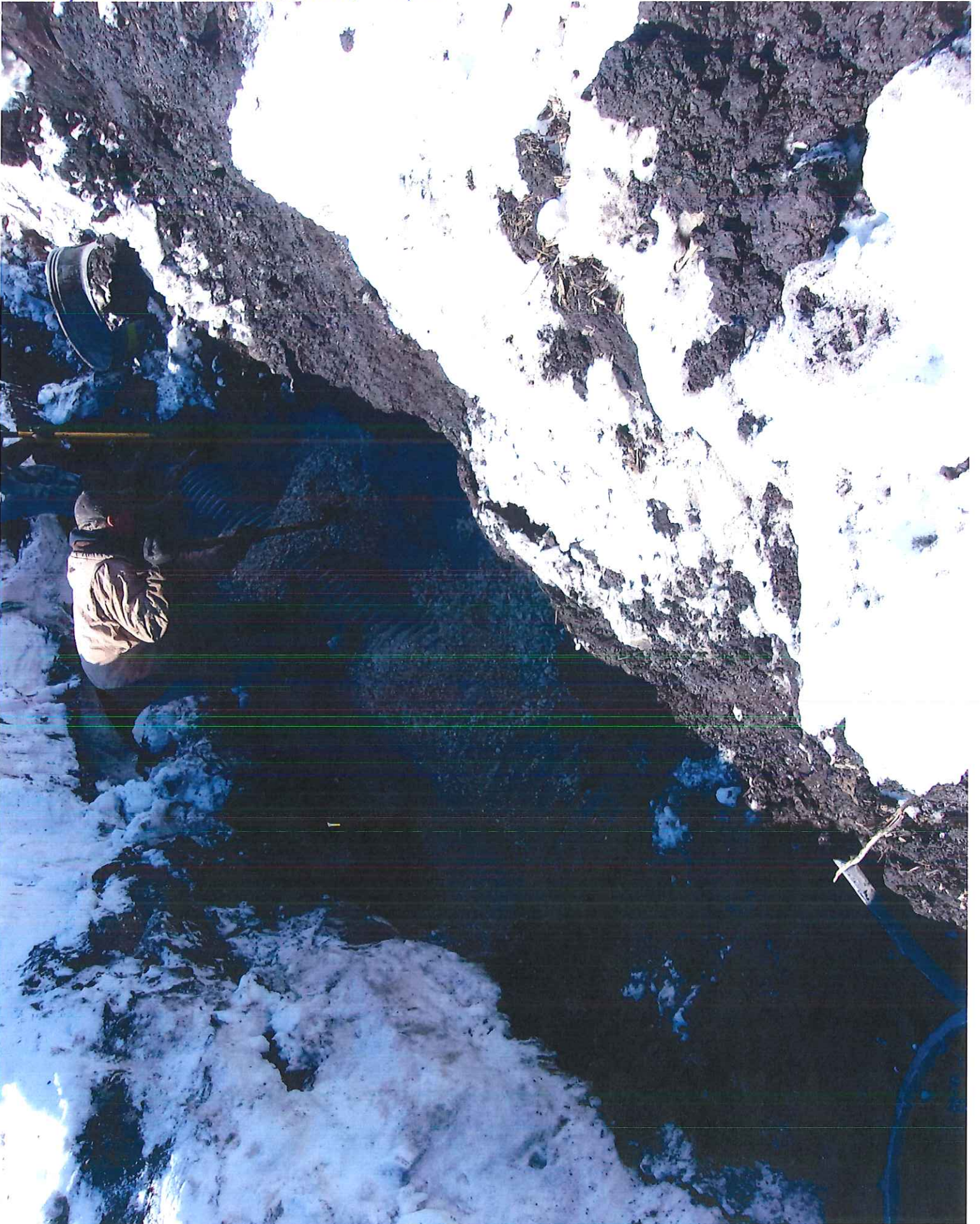
"Chomping" Rock Around HOPP Pipe
